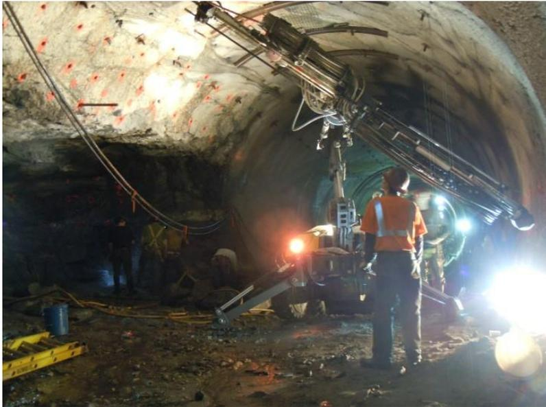
Cross passages between tunnel tubes will be excavated through controlled drilling and blasting (2 weeks per cross passage)
