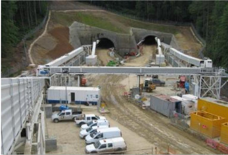
Enclosed conveyor for spoils removal, mufflers and baffles on equipment
