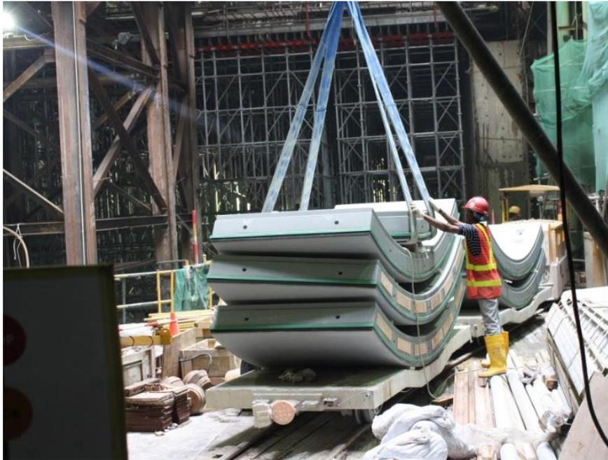
Tunnel will be lined with concrete rings
